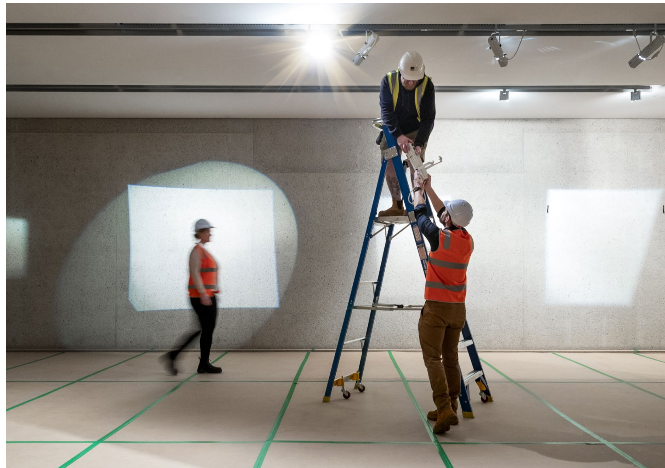
The National Gallery is undertaking a replacement of end of life gallery lighting to LED gallery lighting system to improve energy efficiency.
