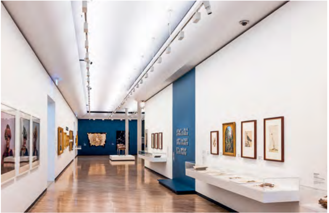
A new LED lighting track and integrated uplighting in Gallery 21
