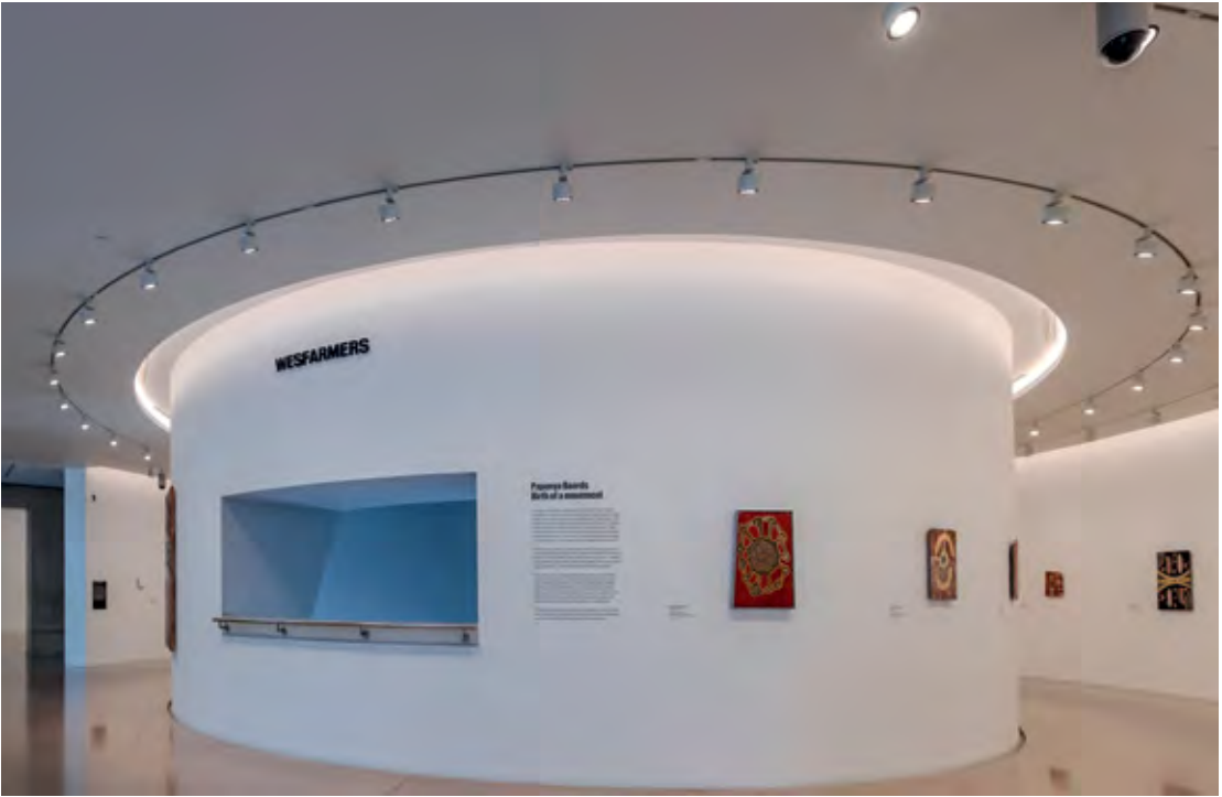
New LED lights and circular lighting track in Gallery 1
