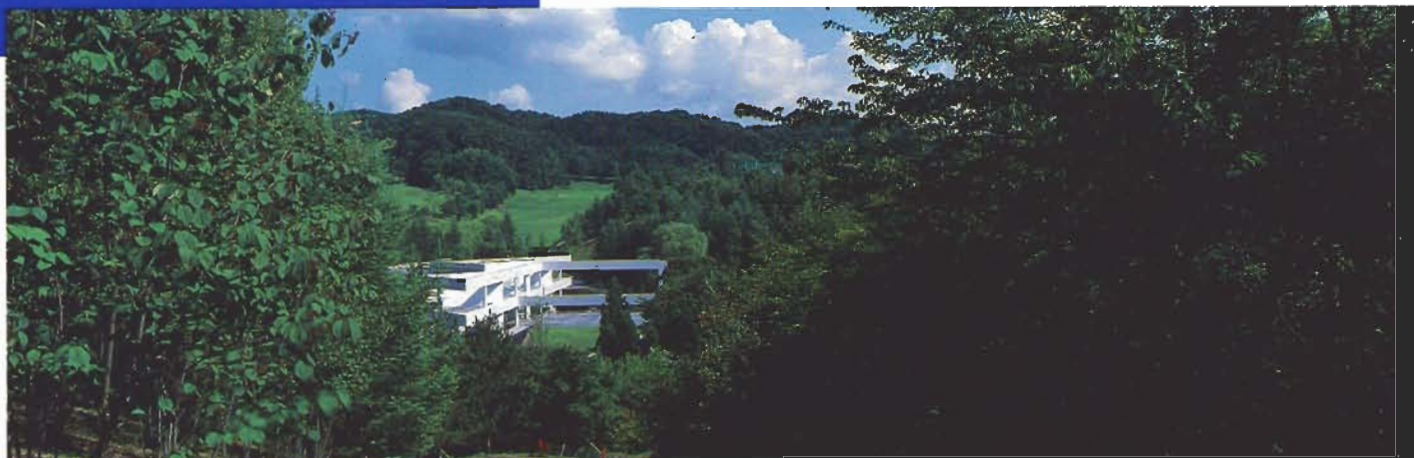
Aerial view of CCGA & TGAC from the northwest
