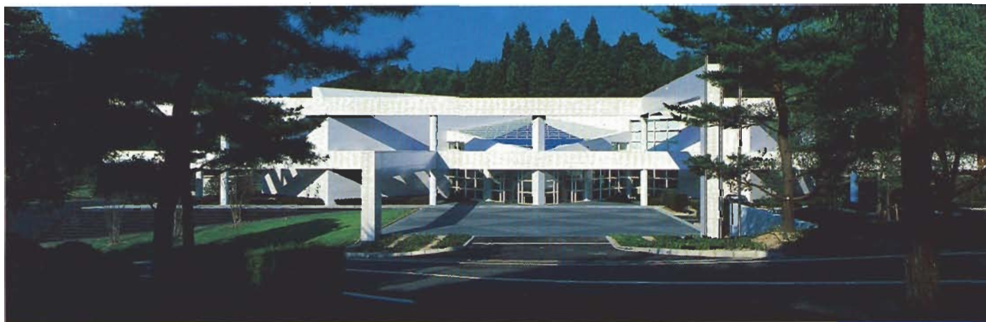
Front of building
