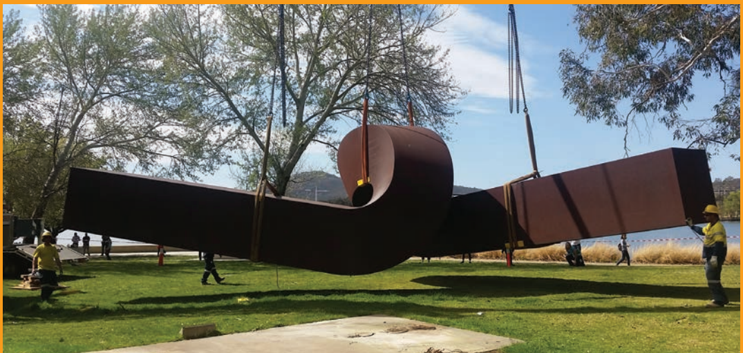
Clement Meadmore's Virginia 1970 being lifted from its old foundation.
